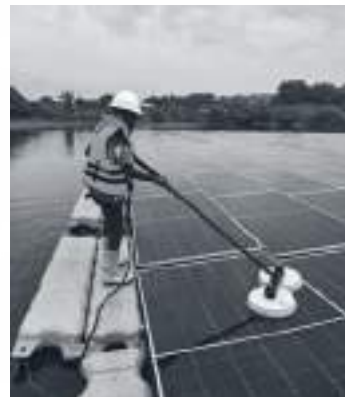
Preventive Maintenance Activity – Photovoltaic Module Cleaning Activity and Photovoltaic String Health Checking
