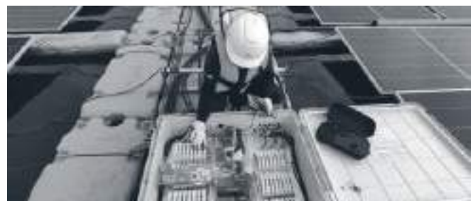
Preventive Maintenance Activity – Photovoltaic Module Cleaning Activity and Photovoltaic String Health Checking
